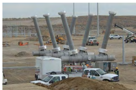
Transmission lines under construction at the Hemingway substation.
