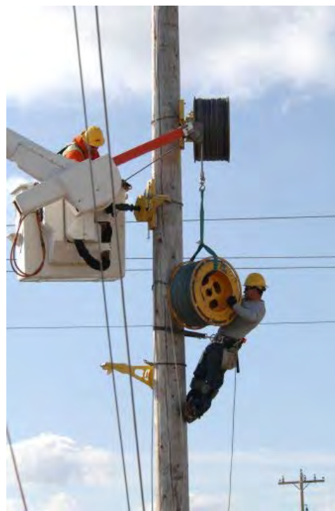
Idaho Power linemen install upgrades.
